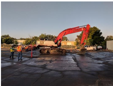
Long reach excavator
